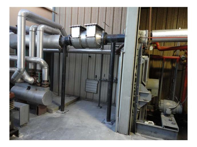
Figure 15: New Catalyst Installed, prior to reinsulation of piping and wrapping catalyst with the manufacturer's furnished removable insulating blankets.
