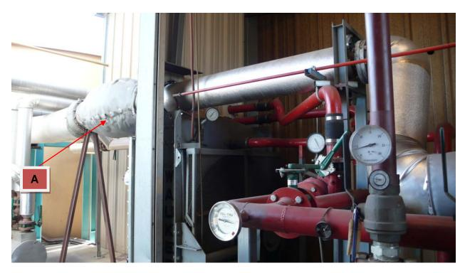
Figure 7: Original exhaust piping viewed from engine toward catalyst (A).
