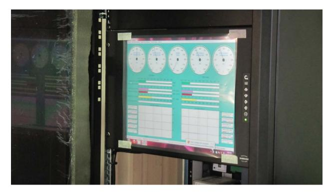
Figure 13: Large, flat panel display allows monitoring of the position, settings and inputs to both valves. The software also logs data for later retrieval and analysis if needed. Data is presented numerically as well as graphically via dials, bar charts and a strip-chart like display
