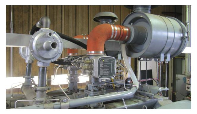
Figure 12: View of reconfigured Fuel System and EGC4 installation.
